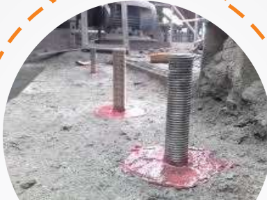
Grouting in J Bolt
